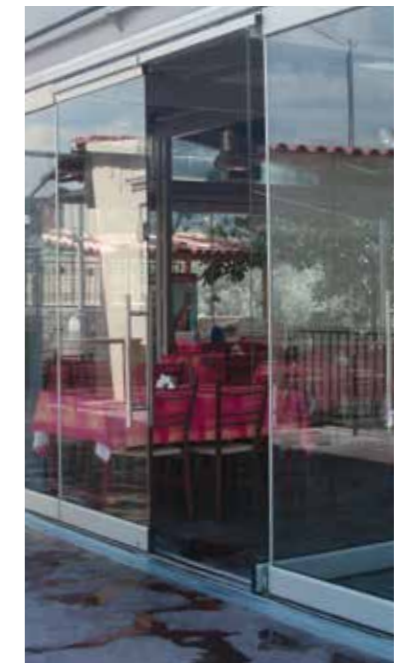
PR200/SOC PANEL SWING - SLIDING DOOR PANEL WITH OVERHEAD CONCEALED DOOR CLOSER IN INTERMEDIATE SECTIONS OF OPENINGS (PR200/ SOC).
